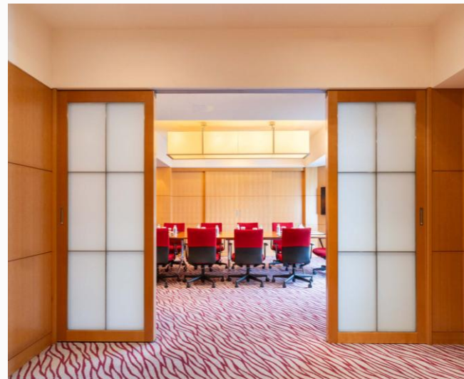
Partition (Openable / Closeable) Opening Width: H2160 × W1500mm
